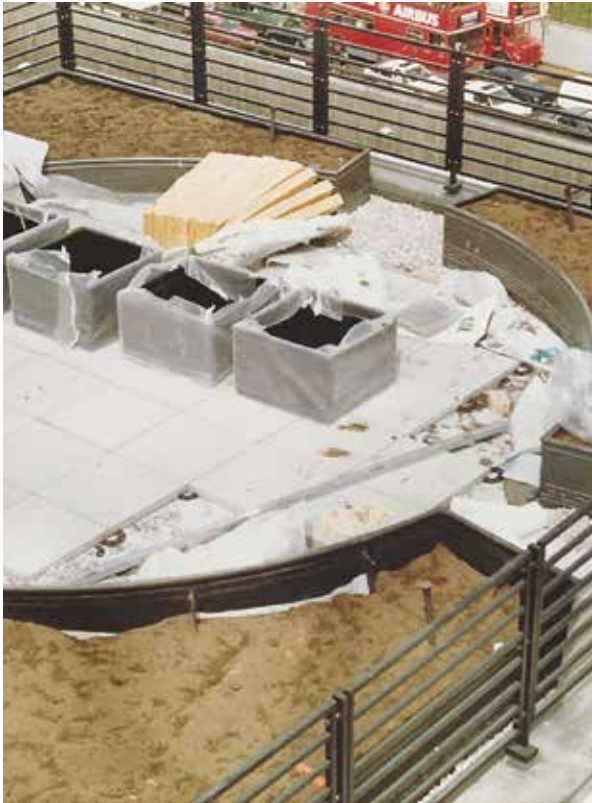
Lanesborough Hotel large bespoke planters for roof terrace
