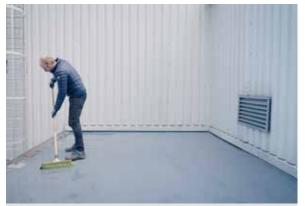
Before starting the installation, clean the roof and check the waterproofing membrane for root resistance and potential defects. In case the roof also requires a roof edge, install the ND KL Separation and Roof Edge Profiles.
